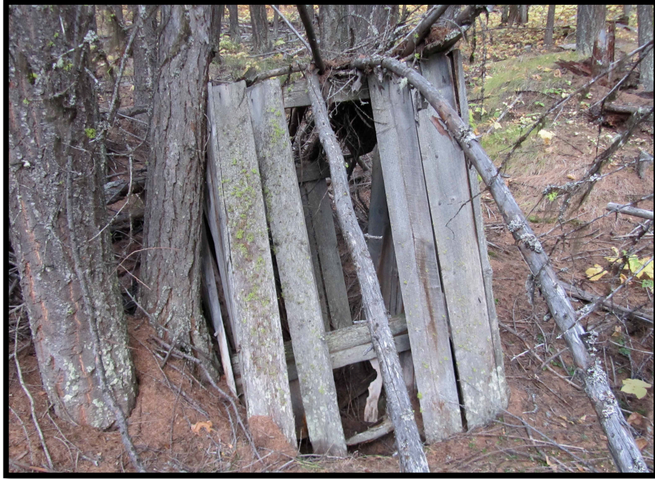
Figure 4.19: Feature 381 prior to removal of floorboards and trees, facing south.
