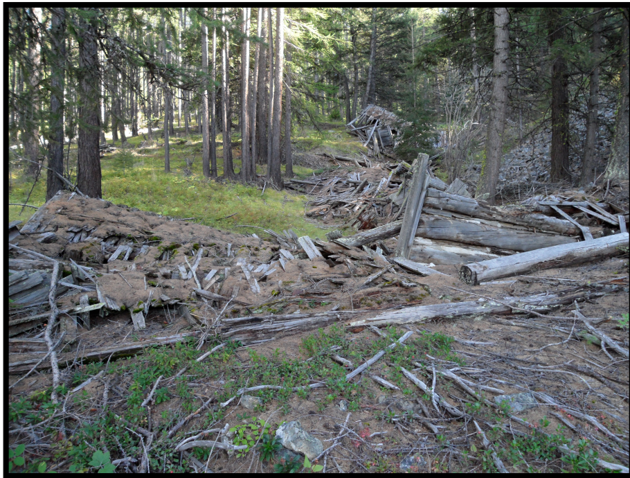
Figure 2.1: Comet site overview from the northwest corner showing the collapsed stamp mill and communal dining structure, facing south, southeast.
