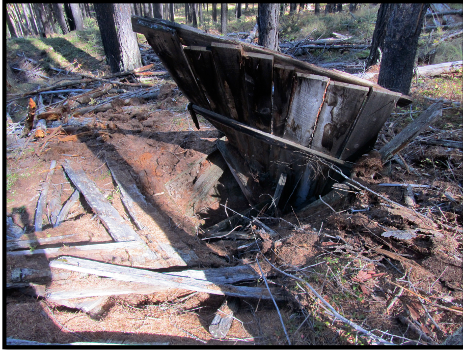
Figure 4.13: Feature 368 (outhouse) prior to the removal of the structural remains, facing northeast.
